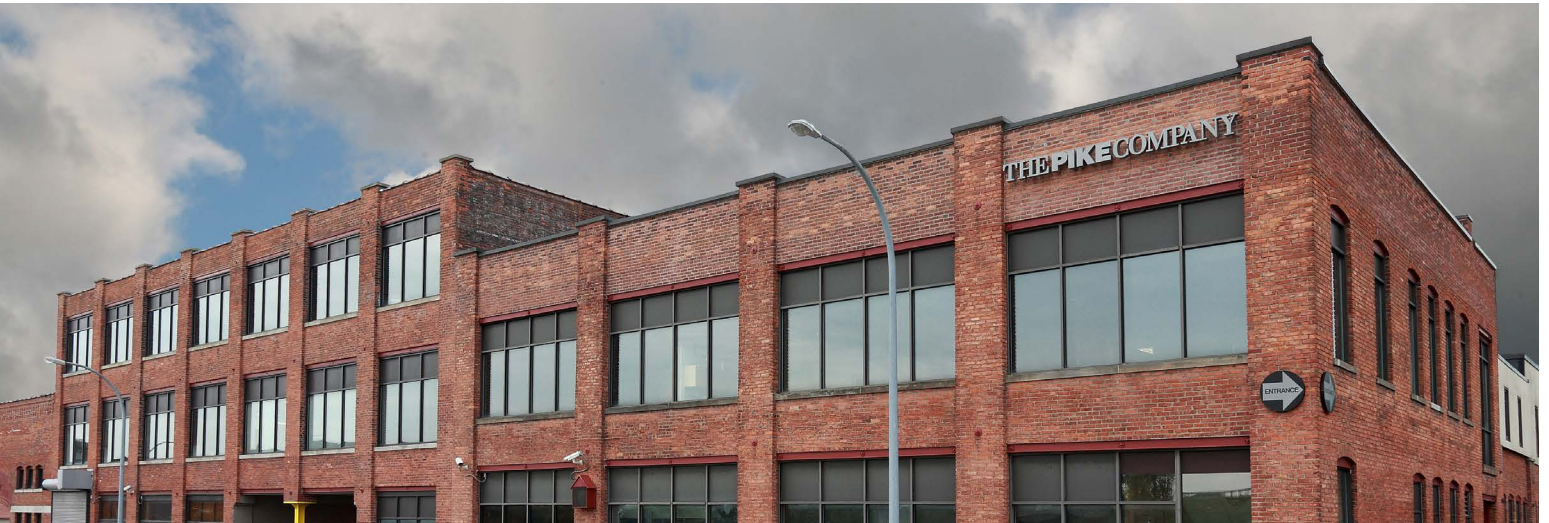
The Pike Company has owned and been headquartered in this historic Rochester building since 1904.
