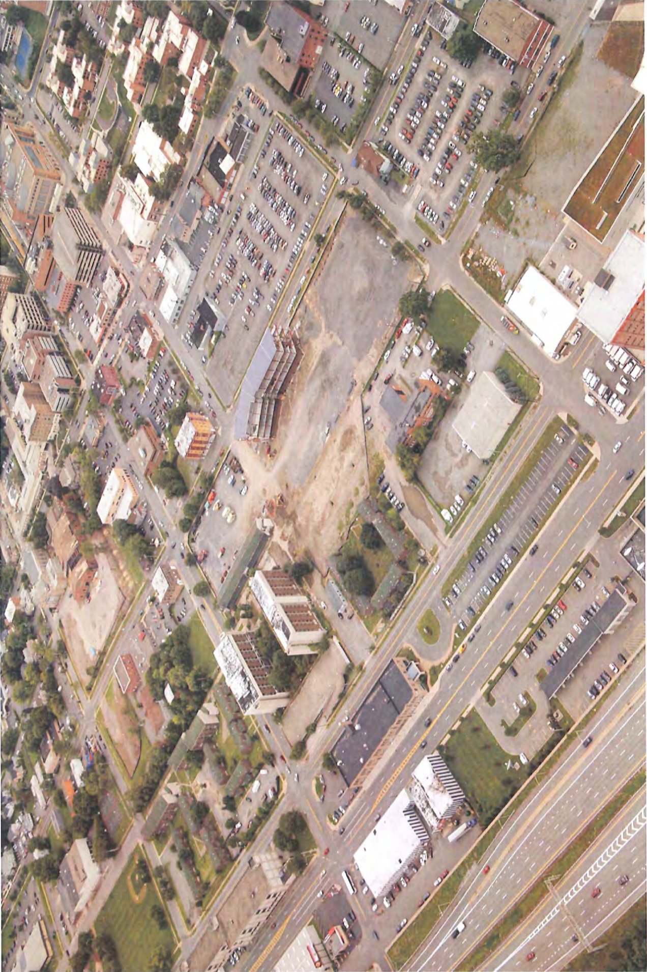
KENNEDY SQUARE – PRIOR TO DEMOLITION
